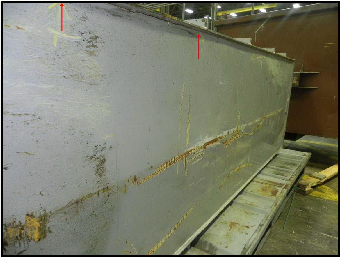
Figure 3: Location of the Crack
