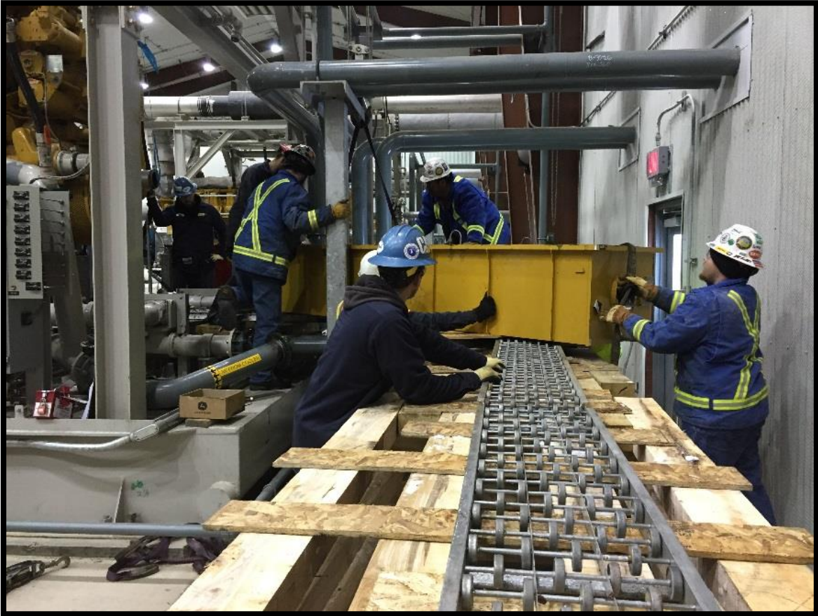
Figure 5: Oil Pan being removed from the Engine via Roller Tracks
