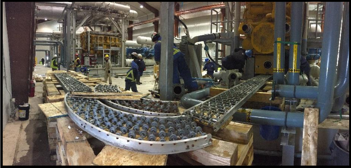
Figure 4: Roller Track used to Remove Oil Pan from Engine
